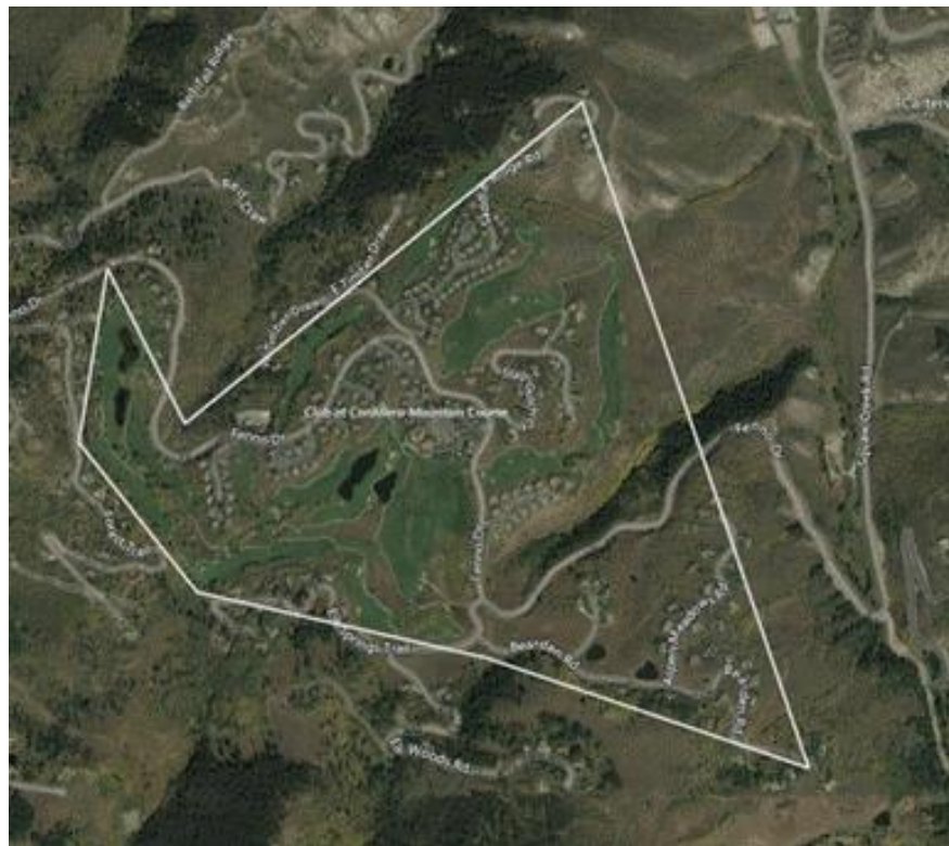
Figure 15: Aerial view of Cordillera, CO community
